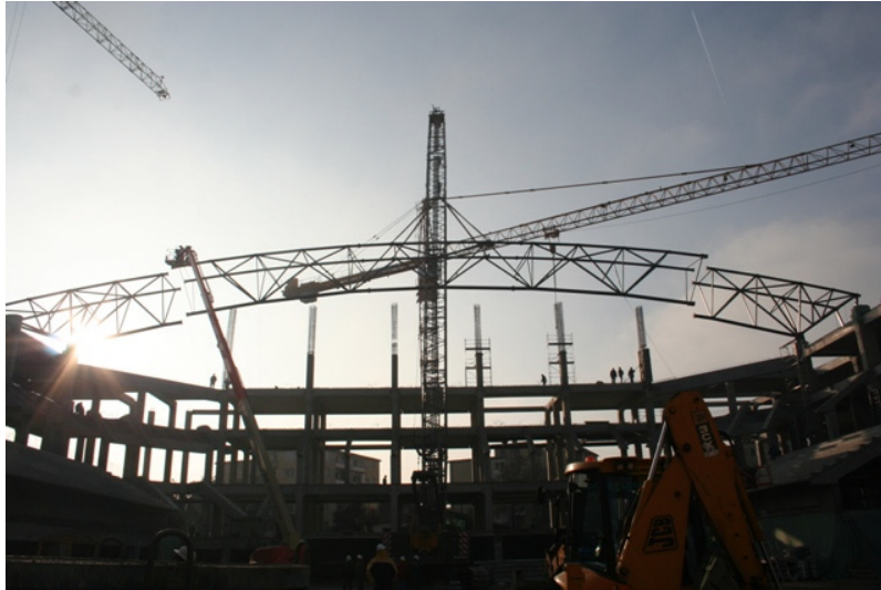
Figure 12: Truss erection on site
