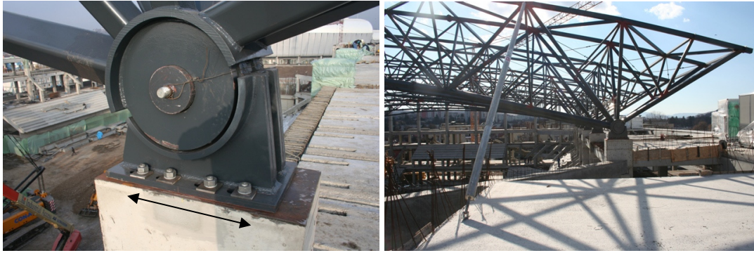
Figure 4: Sliding possibility of the support and view at support level
